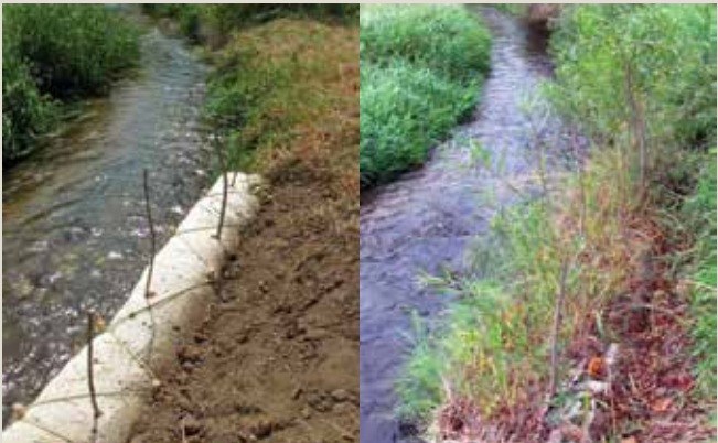
Excelsior fiber erosion control blocks used in a shoreline application with live willow stakes, pictured on the day of installation and three months later. Exterior casing is light in color compared to darker coir logs that can warm water temperatures, which can be detrimental to fish and other aquatic organisms. Functional for 3+ years, but designed to begin biodegrading during the first year as sediment and seed settle into the interior matrix. Also use in other applications such as a replacement for silt fence or for channel filter stations. ©American Excelsior Company
