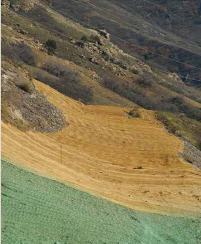
Pipeline reclamation along a steep hillside using both erosion control blankets and a hydraulically applied Bonded Fiber Matrix (BFM). ©Ryan Timoney/Granite Seed
